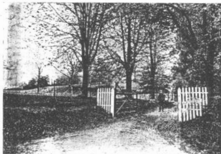
View near the Estate
